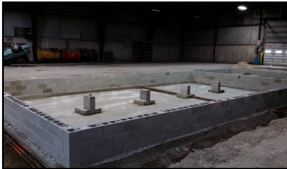
Public Safety Training House Under Construction.
