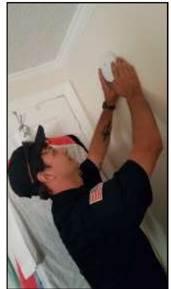
Above: Firefighter Arik Abdullah installing a smoke alarm in Norton Shores.
