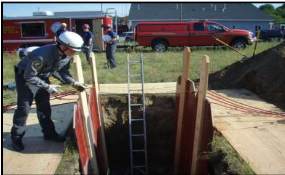
Members from the Muskegon USAR Team practice shoring up the walls of a simulated earth collapse
