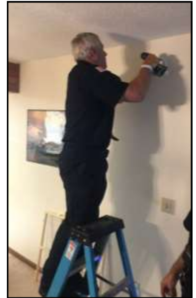
Above: Firefighter Driver Mark Konecny installing a smoke alarm.
